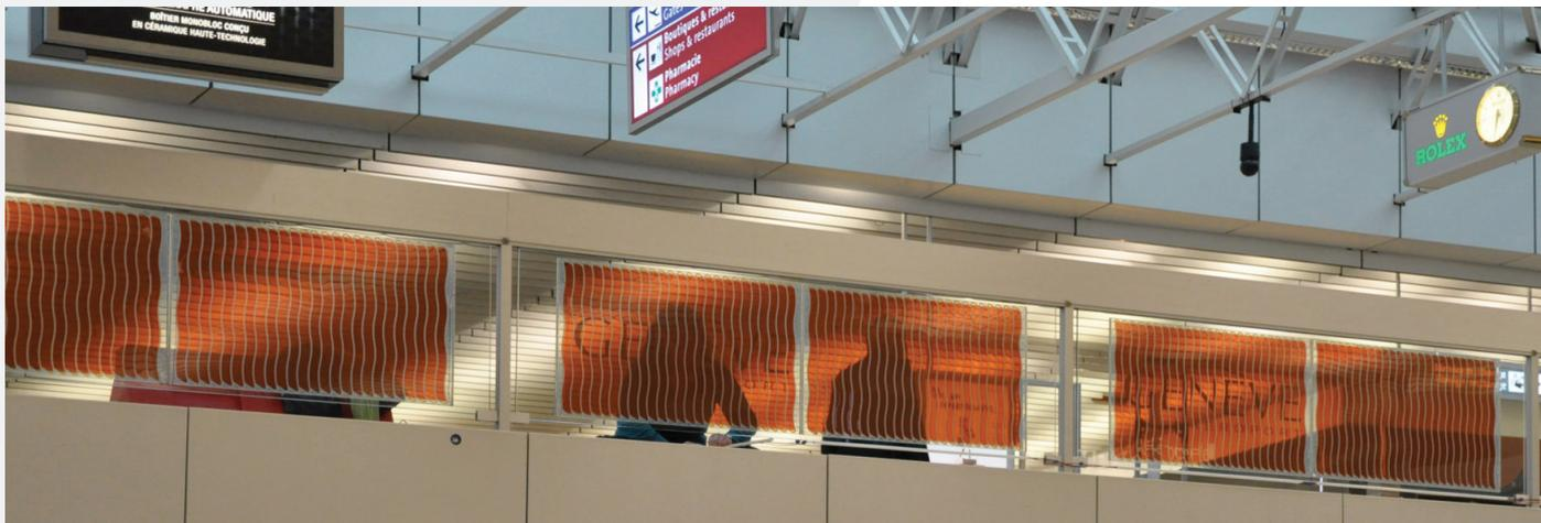
*During the large-scale pre-industrialisation phase, glass2energy (g2e) will exploit the potential of its technology with a photovoltaic balustrade, which has been installed in the area situated in front of the check-in at Cointrin.*
